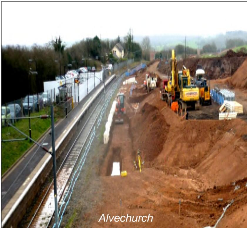
At the heart of the dynamic loop, Alvechurch station will have a second platform (footings are already in place), enabling bi-directional working, whilst both trains simultaneously call at the station. The enhancement will create greater service robustness, whereas at present, any Redditch bound train running irretrievably late, will likely be terminated at Barnt Green, so as not to inhibit single line working through to Alvechurch and Redditch.
