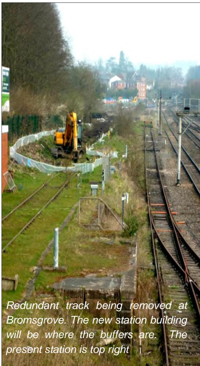
*Redundant track being removed at Bromsgrove. The new station building will be where the buffers are. The present station is top right*
